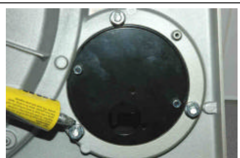
Applying glue to bolt threads
